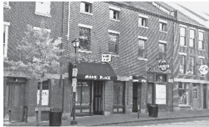
A recent fire at 416-420 Fore Street, in Portland's Old Port, was caused by an improperly installed hot water heater.
