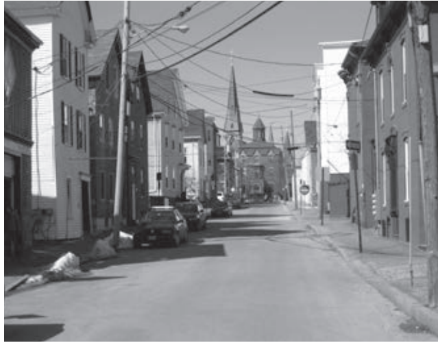
Hampshire Street retains its historic residential scale, and mix of single and multi-family houses.
