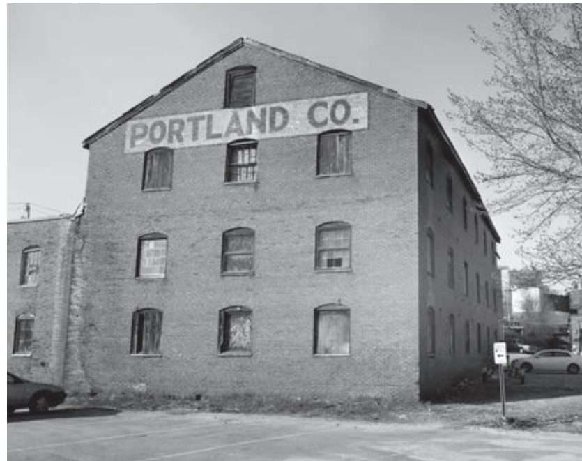
Building 12, built in 1895, was the pattern storehouse for the Portland Company, and introduces the site from the west side of the complex.
