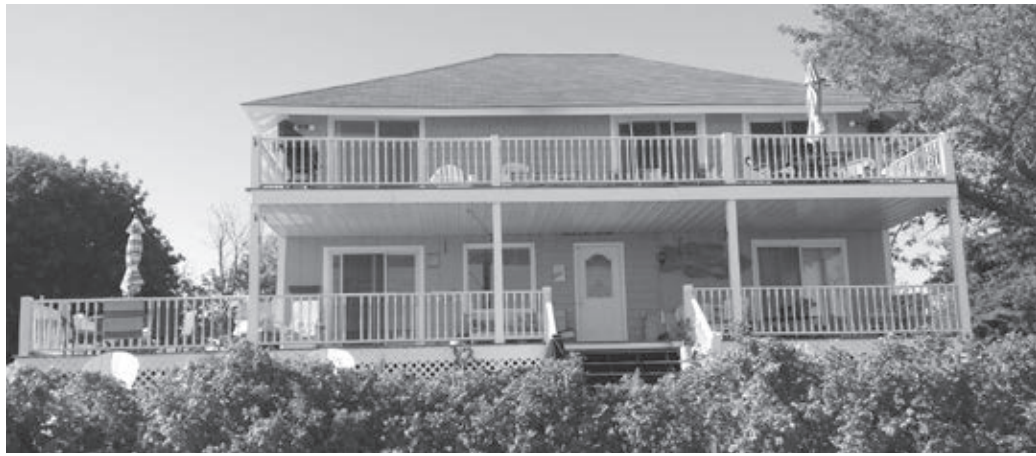
6 Willard Street A former hotel at 6 Willard Street built about 1890 in South Portland retains its form and the former snack bar outbuilding, now boarded up, survives.
