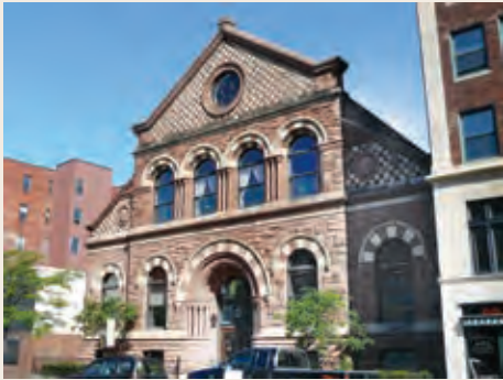
Adaptive reuse of the former Baxter Library (1888) as headquarters for the Via Agency was made possible with federal historic tax credits.
