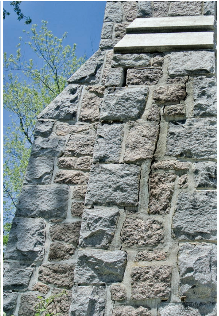
Damaged by use of an inappropriate replacement mortar, the iconic tower of the historic Dunn Memorial Church (1906-1907) in Deering Center needs an estimated $1.5 million to restore its stone exterior.
