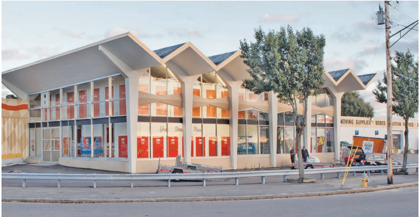
The U-Haul building was a showpiece for Portland Motor Sales, Maine's largest Ford dealership, when it opened in 1963. Today, it is vulnerable to redevelopment as East Bayside evolves as an in-demand location for brewers and distillers and dense residential development.
