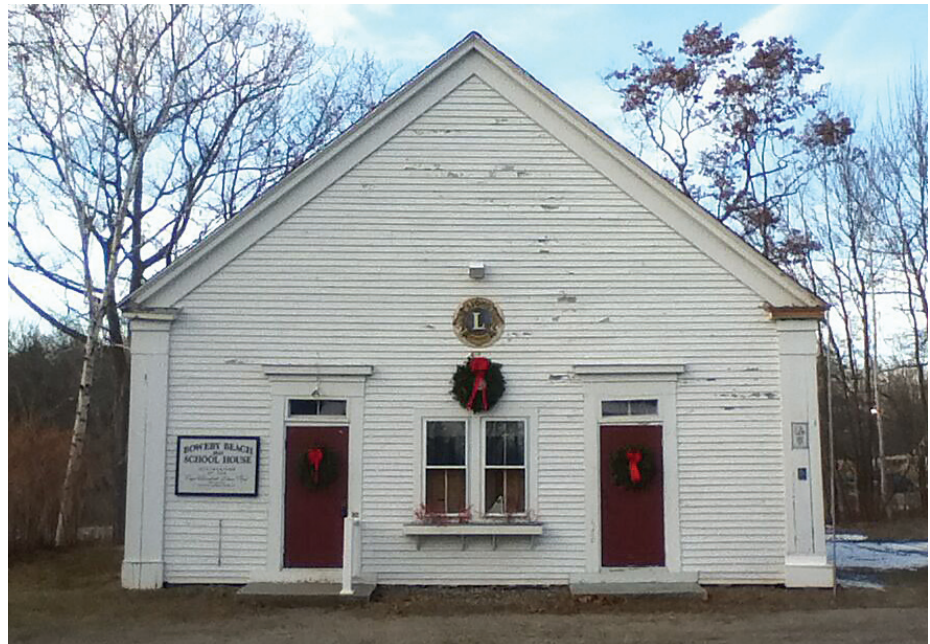
The one-room former Bowery Beach School (1855) needs funding to repair its wooden structure, exterior siding and details.
