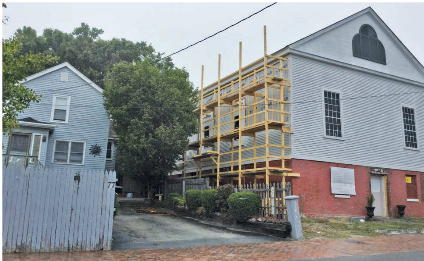
The Abyssinian Meeting House was the center of an African American residential neighborhood off Portland's India Street, including the Abraham Niles House (1844) at left.
