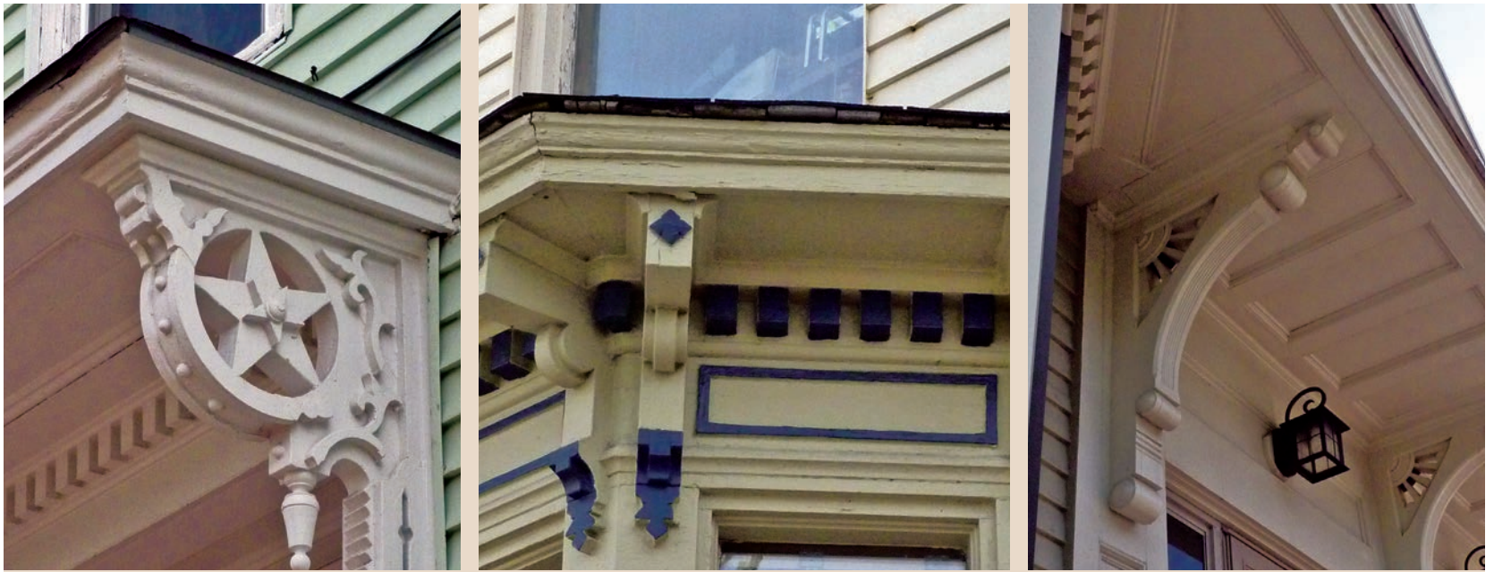
Examples of door hoods, bracket ornaments, and denticular details that are indicative of development on Munjoy Hill following the Great Fire of 1866 and give the neighborhood buildings their distinctive character.
