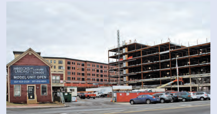
Hobson's Landing at the former Rufus Deering Lumber Co. takes shape.
