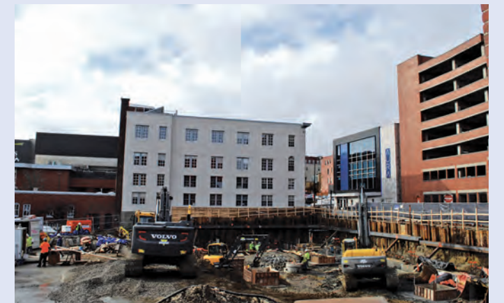
Construction of the Free Street Apartments is underway.
