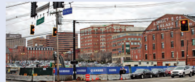
Center Street Hotel construction begins.
