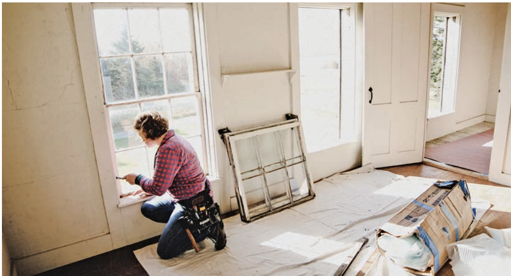
Removing windows for restoration at the Hathorn-Olson House
