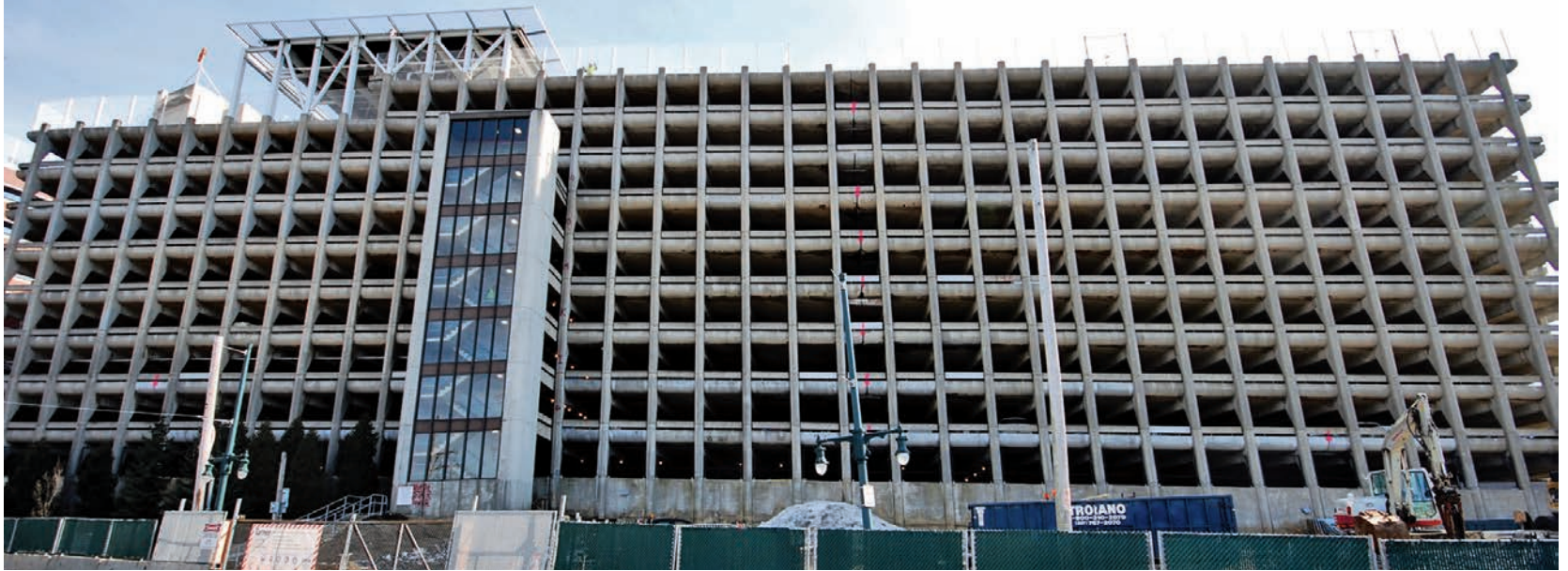
Maine Medical Center's c1970 brutalist parking garage was demolished this year.
