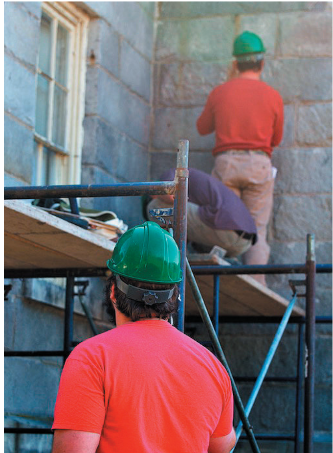
Masonry students work on the Kennebec Arsenal.
