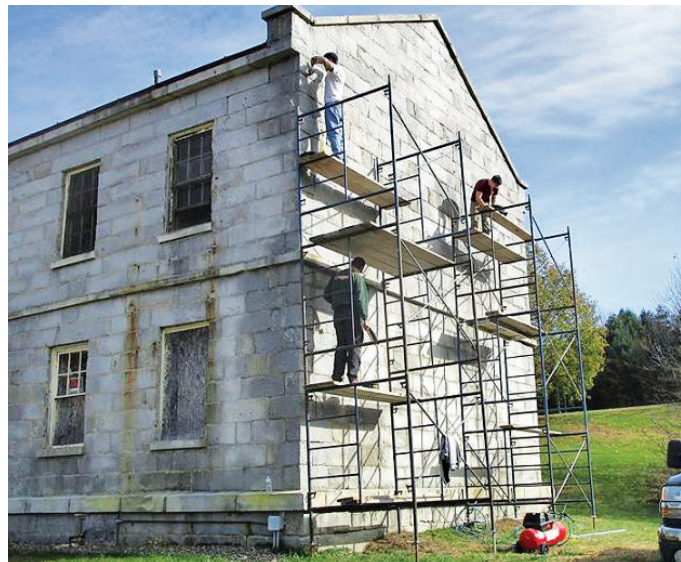
Students on site repointing the barracks at the Kennebec Arsenal.
