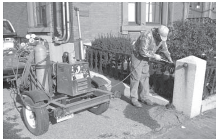
Tim and Gretchen Greene of StandFast Works Forge donated their time repairing the fence at Landmarks' Safford House headquarters. The Greenes, who are based in Parsonsfield, were working in Portland on another project and noticed the poor condition of the fence. They removed loose pieces and created molds to cast replacements, and repaired broken links to make the fence sound. Landmarks thanks Tim and Gretchen for their generous donation!
