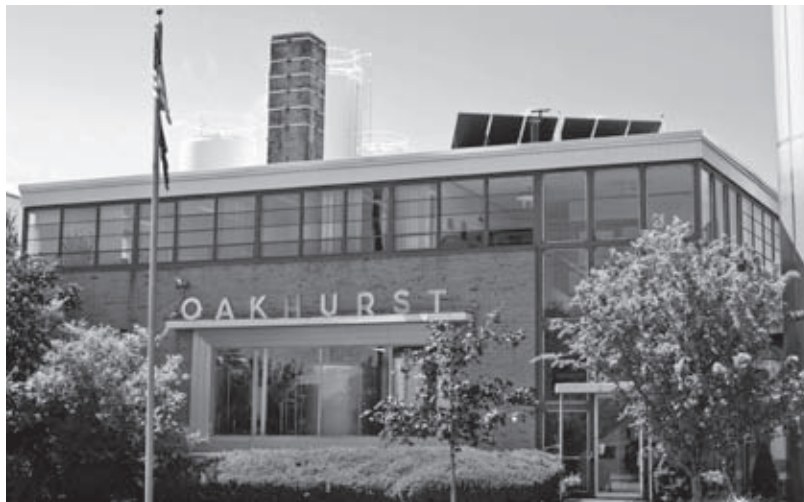
The Oakhurst Dairy (1951-53), a fine example of the International Style, features a large window that reveals the storage tanks inside.
