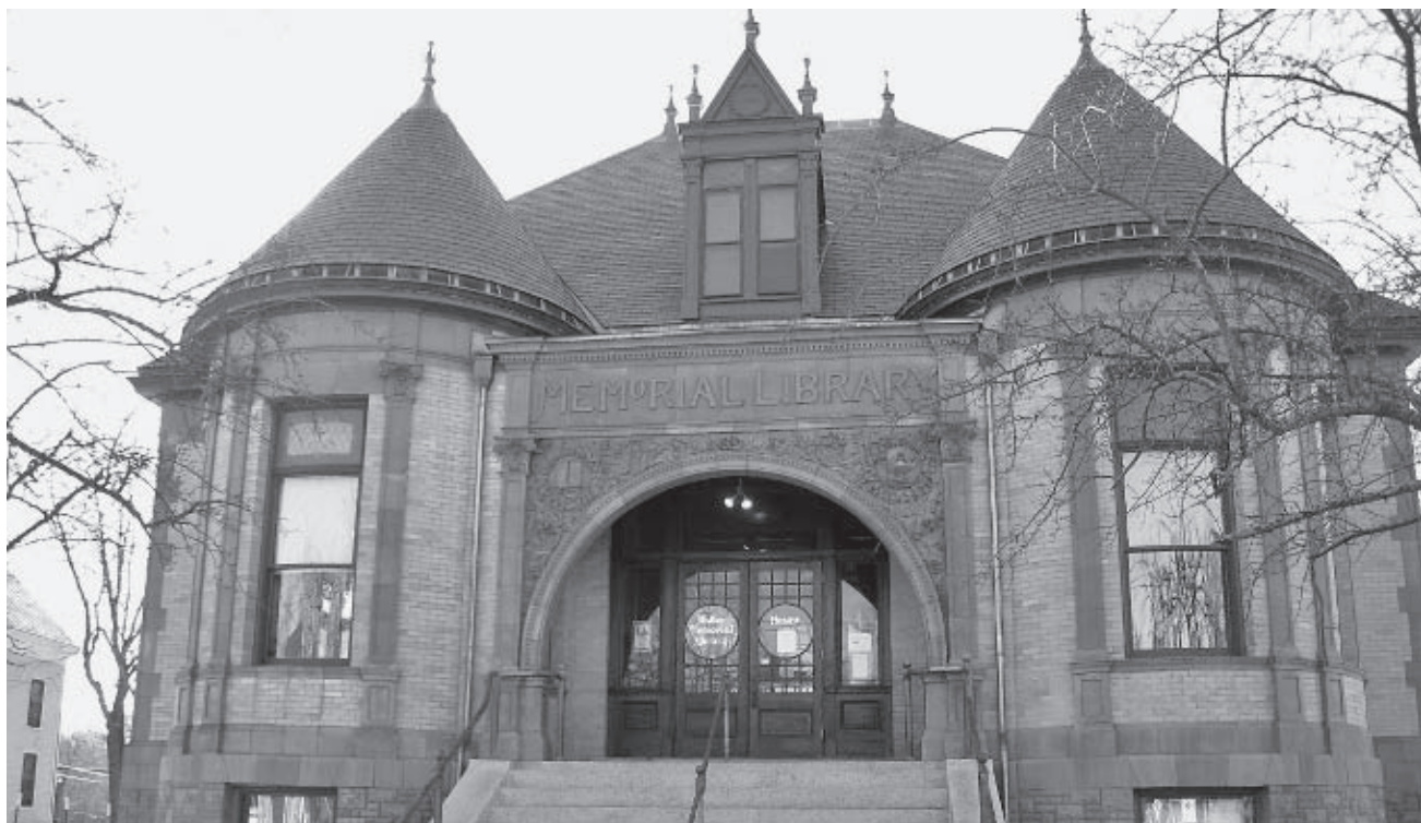
The library's slate roof and decorative finials were among major restorations done by local trade artisans.
