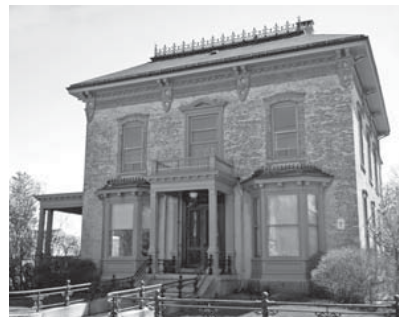
A membrane roof covers the flat part of this historic home's roof, above the decorative grill where it can't be seen.
