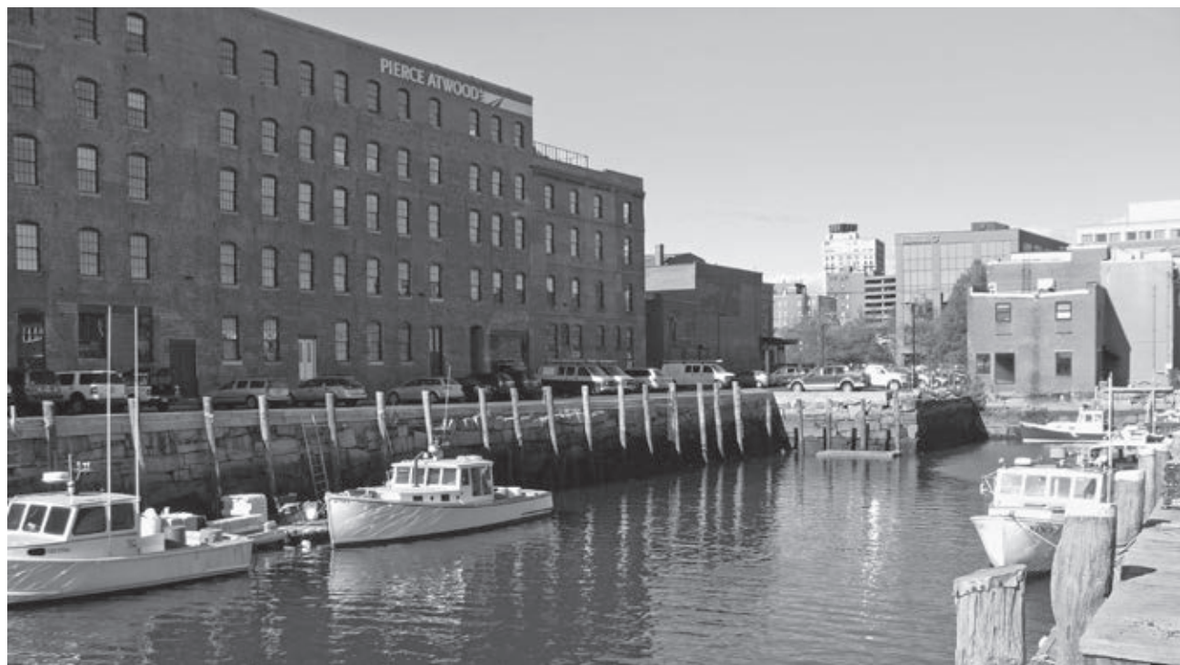
The previously neglected Cumberland Cold Storage/Twitchell-Champlin building (1884-1924) has been revitalized as the new Portland headquarters of the law firm Pierce Atwood.
