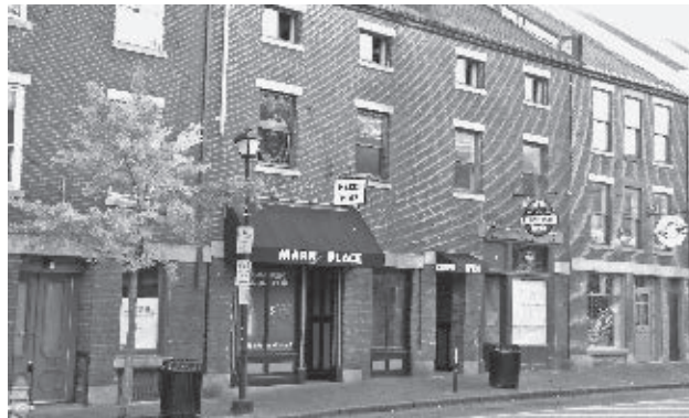
A recent fire at 416-420 Fore Street, in Portland's Old Port, was caused by an improperly installed hot water heater.
