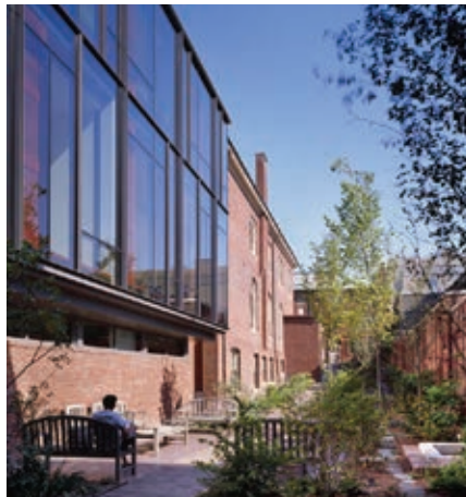
The new Brown Library at Maine Historical Society designed by Schwartz Silver fits well with its landmark neighbors, the Longfellow House and the original library building.
