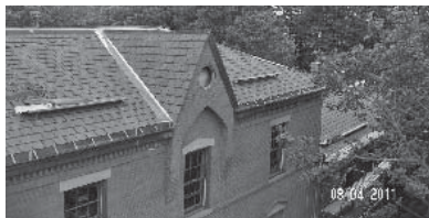
Waynflete H.S. Phase 2 Completed Aug. 2011
