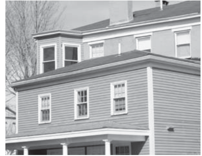
Windows are a major source of energy loss in an older home; storm windows can make a significant difference.
