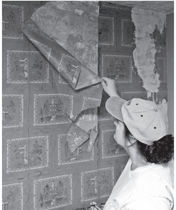
Potentially facing multiple layer of paper, vinyl papers or painted over wallpapers, removal calls for patience and elbow grease more than anything else.
