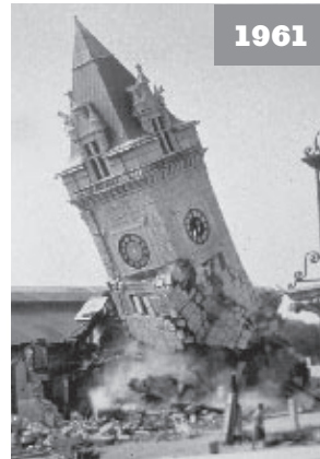
UNION STATION DEMOLITION
